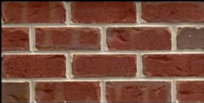
413FL Burnt Chimney Oversize
